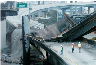
Fig. 1. Bridge collapsed after fire [12]
