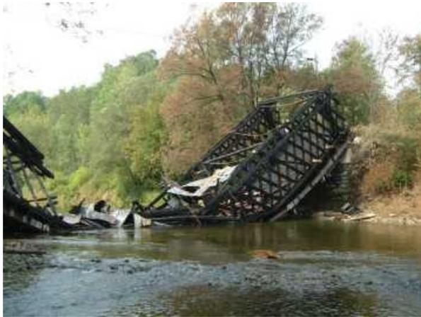
*Fig. 1.* Bridge collapsed after fire [12]
