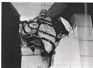
Fig. 1. Large drift and shear failure of a column due to thermal expansion of floor [2]
