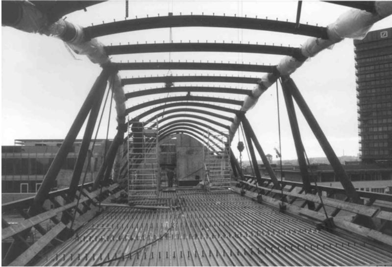
Fig. 2. Primary structure of the 7<sup>th</sup> floor office space
