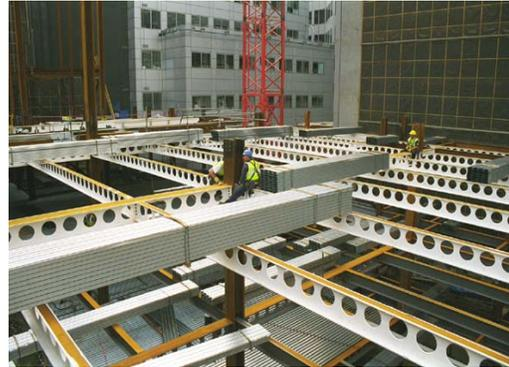
*Fig. 1. Use of cellular beams in buildings*
