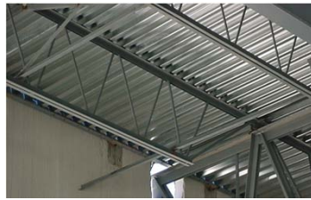
Figure 1. A steel truss supporting the roof of the structure
