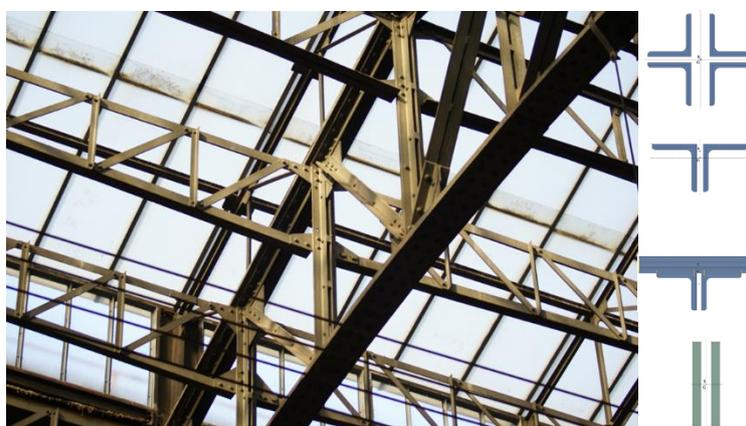
Figure 6-16 The steel structure and typical profiles of the main girder.
