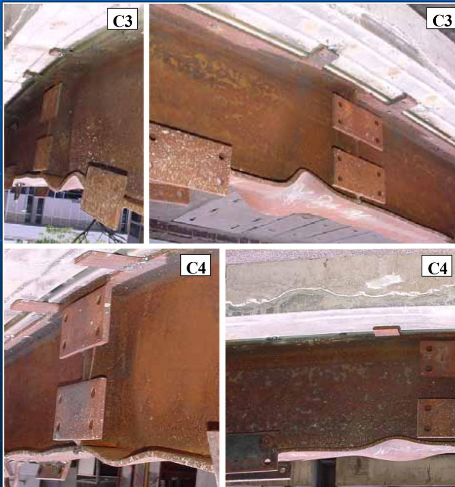
➤ Anti-symmetric local buckling of bottom flange where one side of flange curled up while the other side twisted downwards
