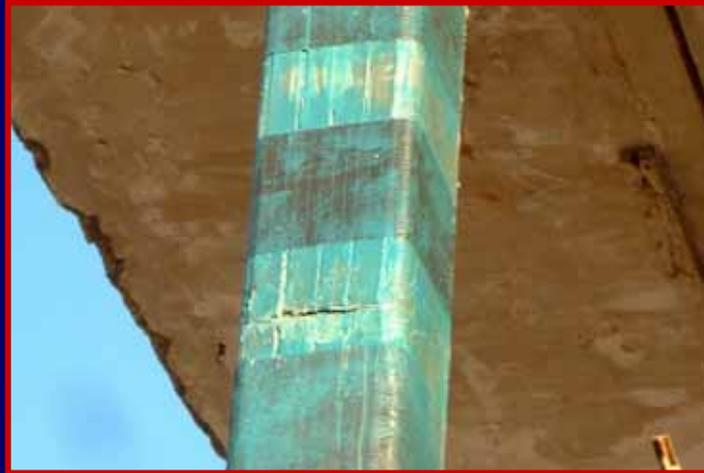
Cracking of beams in torsion
