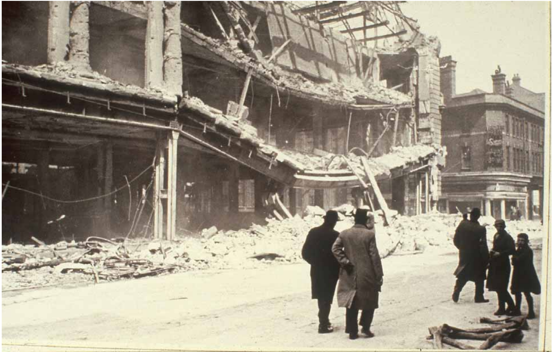
Building illustrating the significant connection rotations developed following bomb attack
