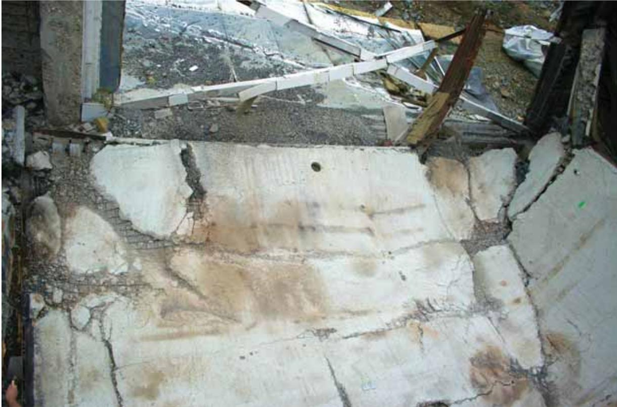
Fig. 8.6 - Edge of the slab affected by the crushing of the concrete
