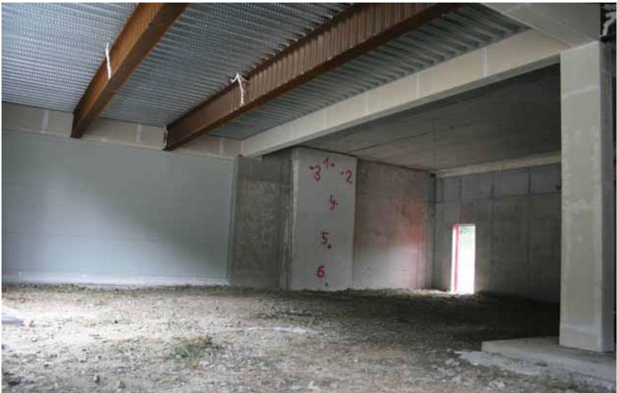
Fig. 1.9 - The east part of the fire compartment before the test
