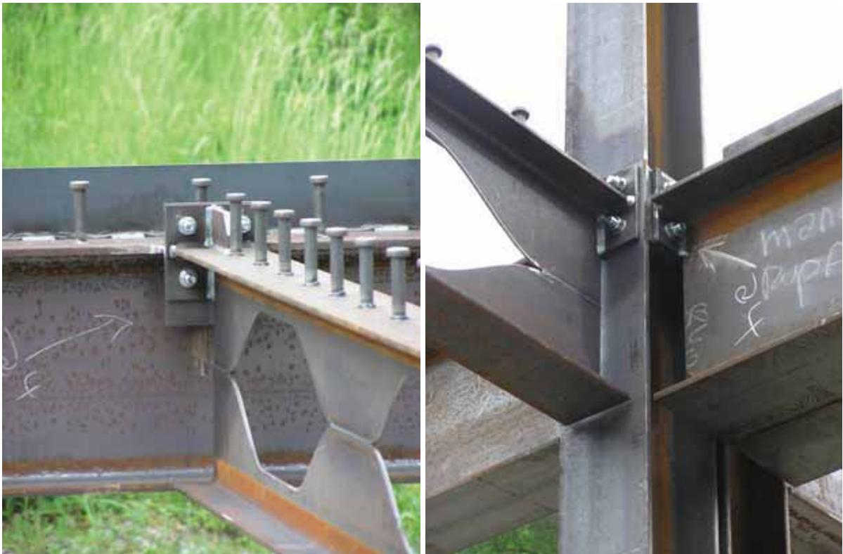
Fig. 1.5 - Connections to the edge beam and internal column
