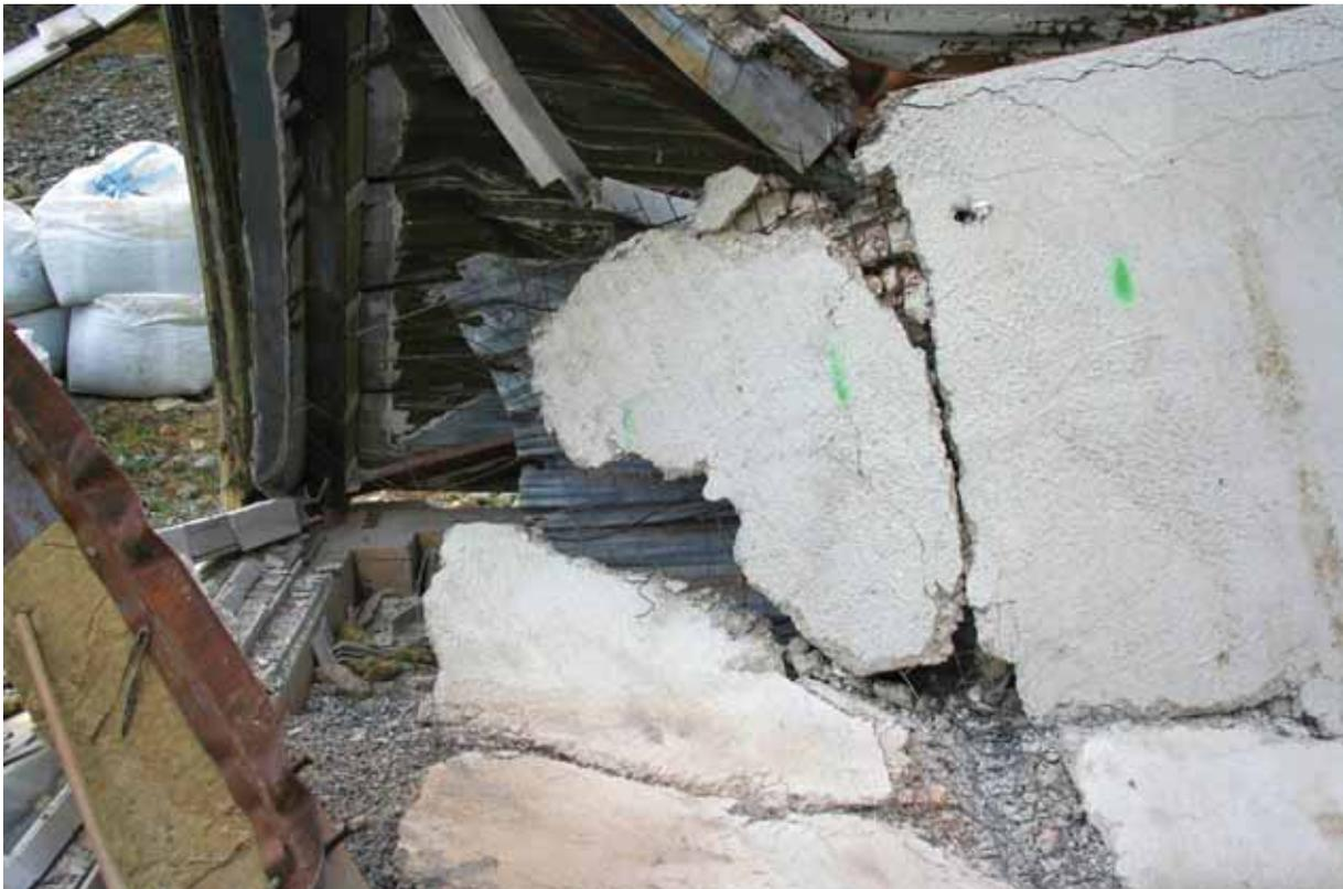
Fig. 8.5 - The corner of the composite slab, where the initial damage began
