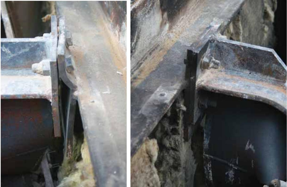
Fig. 8.10 - The cellular Angelina beam to the central primary beam connection on the primary beam after its collapse
