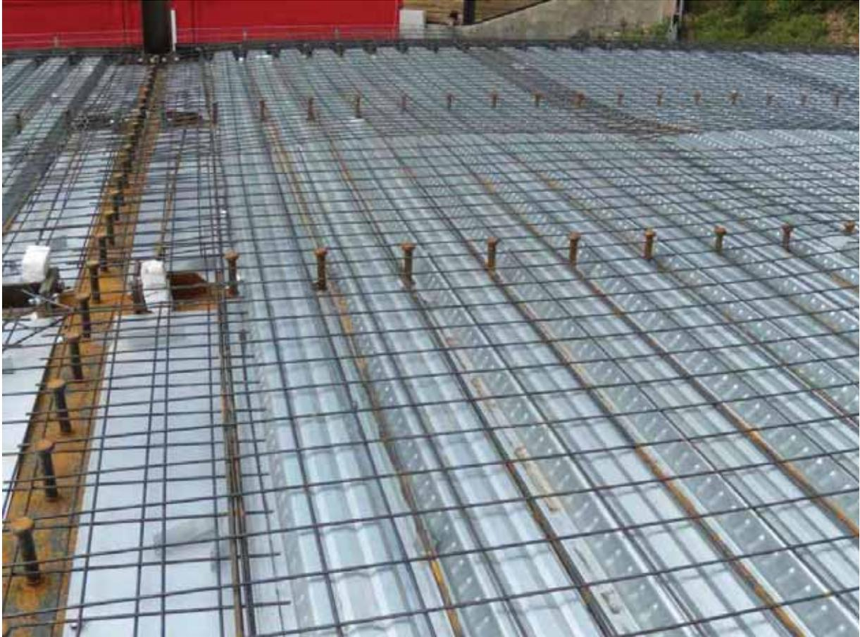
Fig. 1.6 - Connection of the reinforcing mesh on the secondary beam
