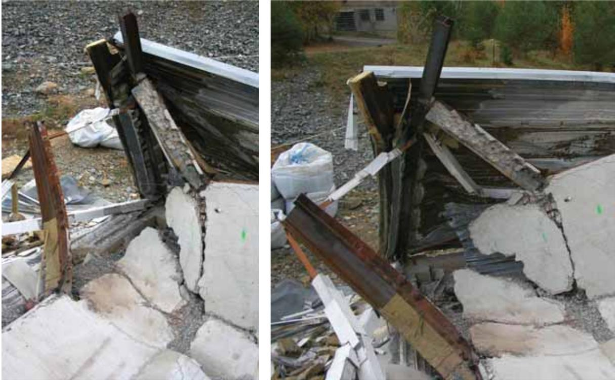
Fig. 8.8 - The edge beam in the corner of the slab after buckling
