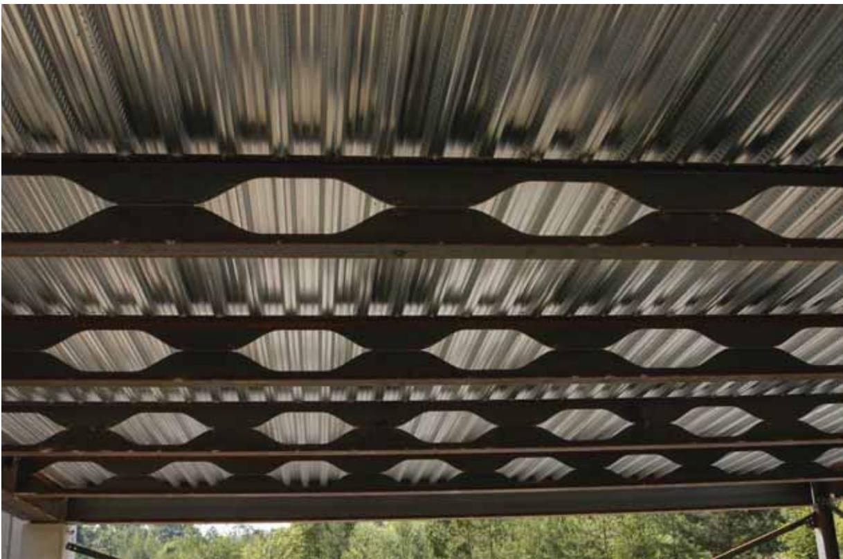
Fig. 1.3 - Composite slab with castellated beams
