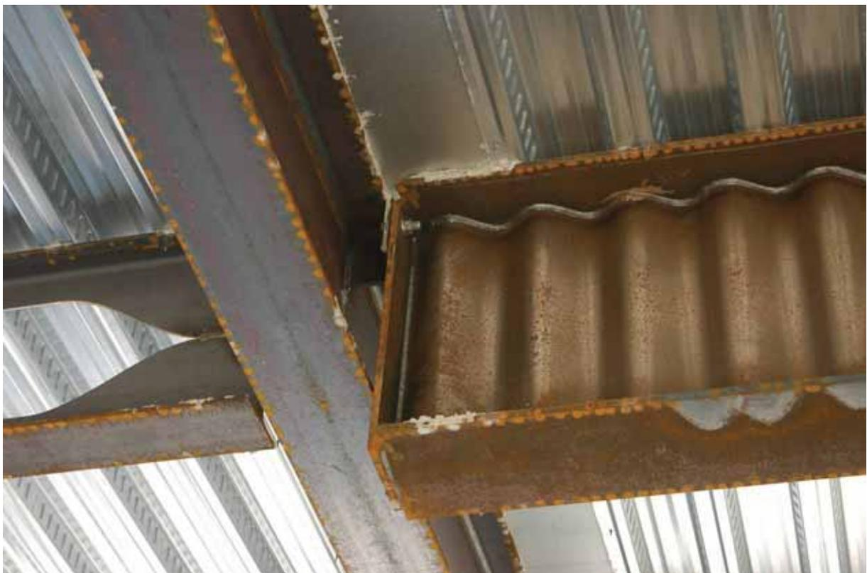
Fig. 1.7 - Connections to the secondary beam
