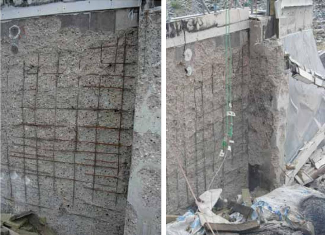
Fig. 4.48 - Loss of concrete in the wall and at the top of the column
