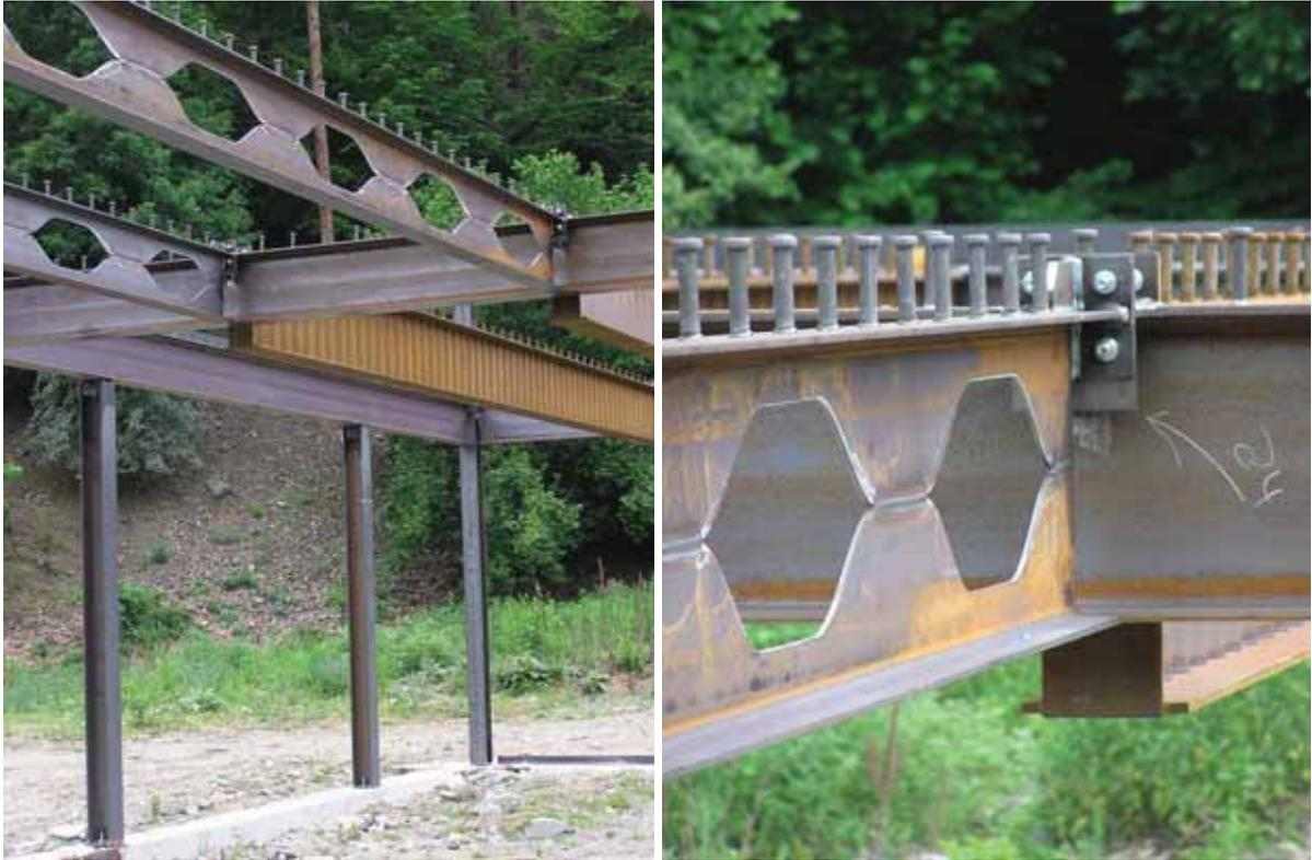
Fig. 1.4 - Connections to the secondary beam
