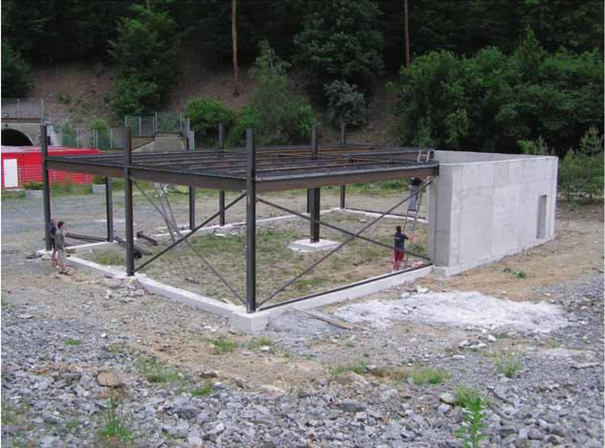
Fig. 1.2 - Erection of the steel structure
