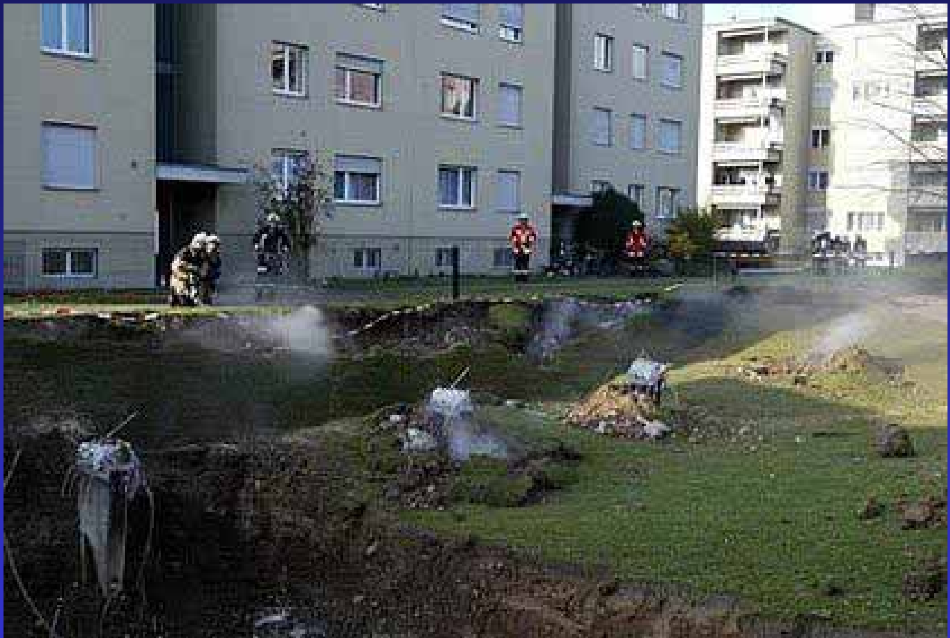
Collapse of an underground car park after the fire has been put down 35
