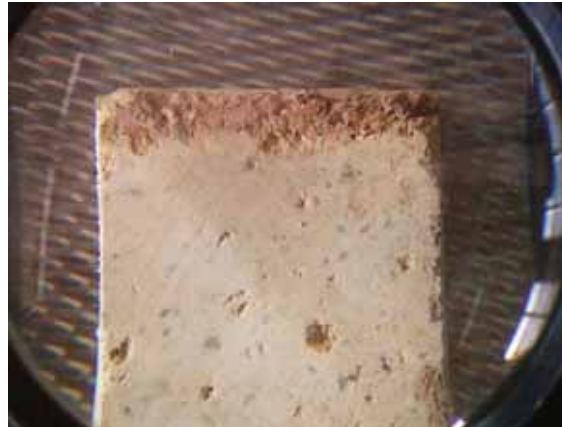
Thickness degraded - 2,95cm
