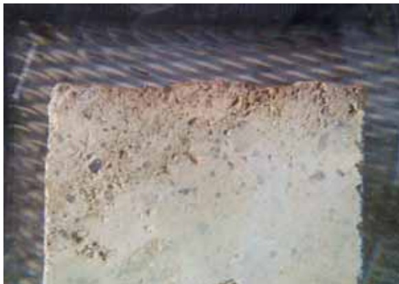
Thickness degraded - 3,56cm
