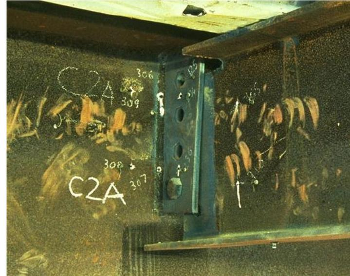
Bolt failure occurred during cooling phase
