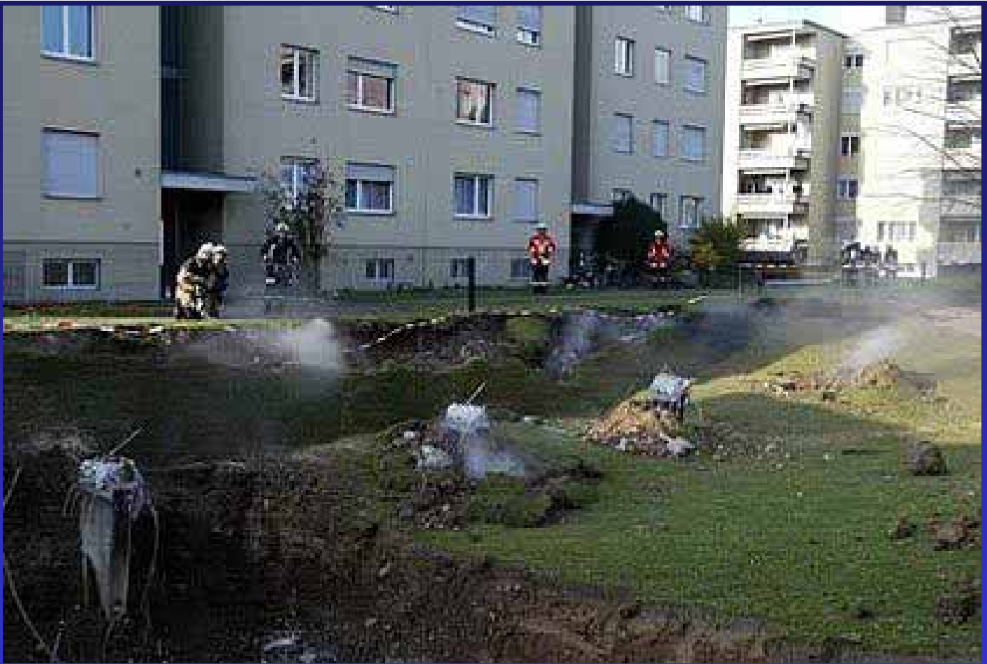
Collapse of an underground car park after the fire has been put down 35
