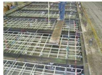
*Figure 8: Slabs reinforcement grids before casting.*
