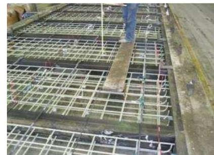
*Figure 8: Slabs reinforcement grids before casting.*
