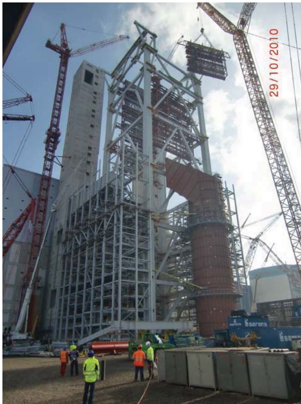
Fig. 19.2 Erection of the main frame of the boiler house (29/10/2010).
