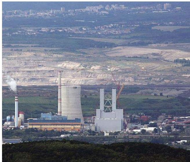
Fig. 19.1 Erection of the boiler house building in power plant Ledvice with two concreted braced towers providing horizontal stiffness.
