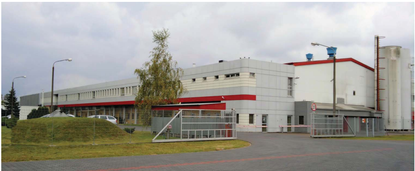
Fig. 21.1 General view of the bakery plant building
