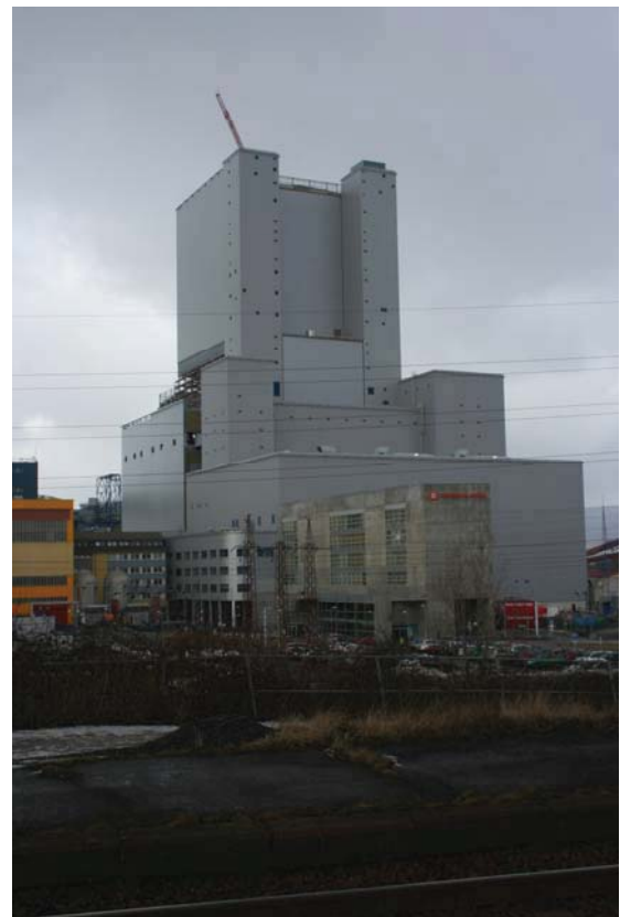
Fig. 19.3 Finalised external structure on the building of the boiler house (13/2/2012).
