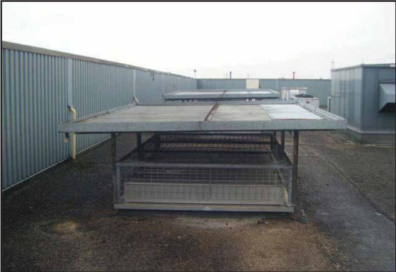
Fig. 13.5 Roof ventilation covers
