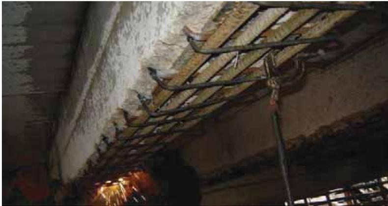
Fig. 30.16 Additional stirrups of beam B2, welded for the existing one.
