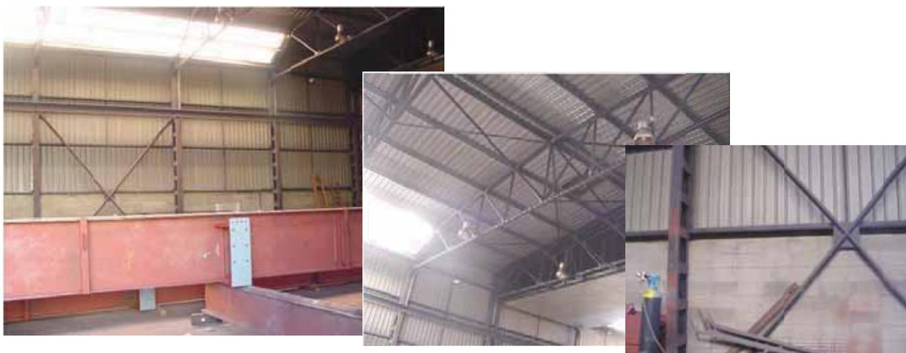
Fig. 20.2 Conventional bracing systems in the walls and rafter
