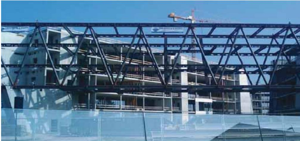
Fig. 3.3 Truss girder spanning over main entrance during construction phase (©hhpberlin)
